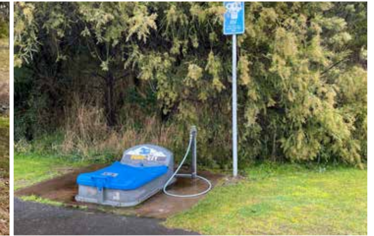
Crookwell Caravan Park RV dump point - positional signage at this location required
