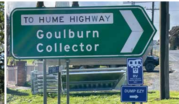
Gunning - ineffective undersized signs
