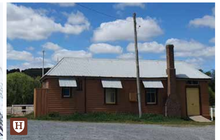
Crookwell Railway Station - no signage. List attraction opening hours on UL Tourism website
