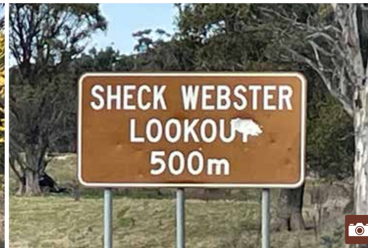
Sheck Webster Lookout - sign damaged, this sign should carry the Australian Standard Lookout symbol
