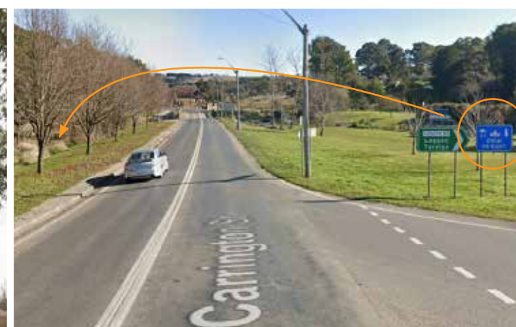
This sign is positioned on the wrong side of the road
