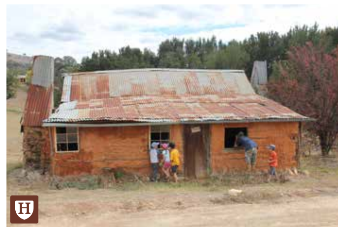
Book Keepers Cottage, Tuena. No directional signage to this attraction
