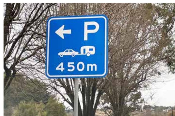
No reciprocal advance warning sign for westbound Goulburn Rd Visitors. Sign too far from decision point
