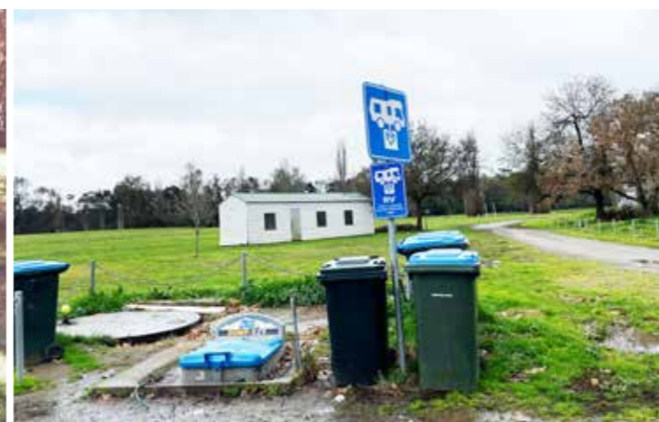
Jugiong RV dump point, no directional sign to this location from Riverside Dr. Dump point area needs to have a proper pad installed.
