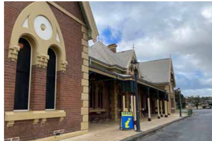
Young Visitor Information Centre - Due to the historical significance of the Young Train Station no large signage can be attached to the building
