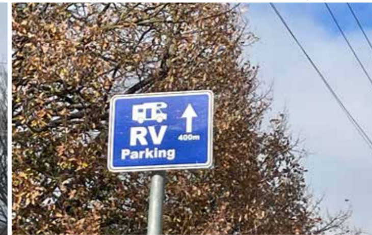
RV parking advance warning signs are too small. As traffic is travelling below 80kph these signs only need to be positioned 200m either side of the parking area.
