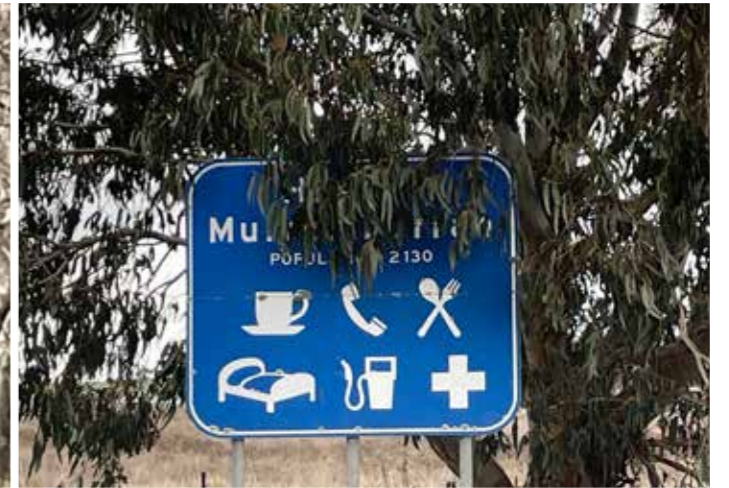
Harden - Advance warning signage overgrown
