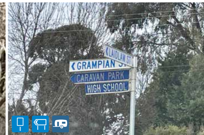
This important turn-off should have a chevron directional sign at this important intersection with advance warning signs positioned 200m either side of this intersection (see example page 37)
