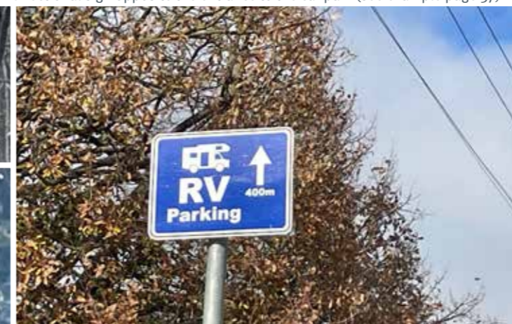
RV parking advance warning signs are too small. As traffic is travelling below 80kph these signs only need to be positioned 200m either side of the parking area.
