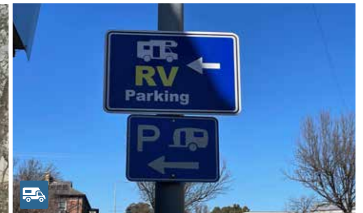
Yass - signage too small, use non standard design, non AS symbol (RV)
