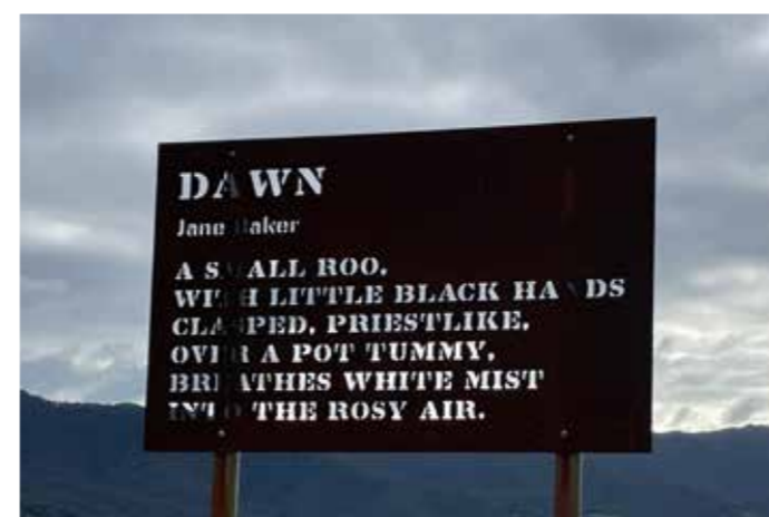
Wee Jasper Rd - Laser cut sign panels ruined by poor placement of sign posts
