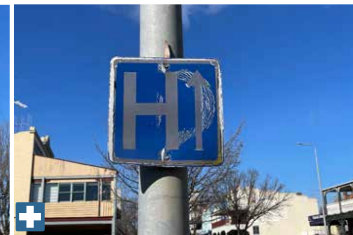
Old out date hospital sign
