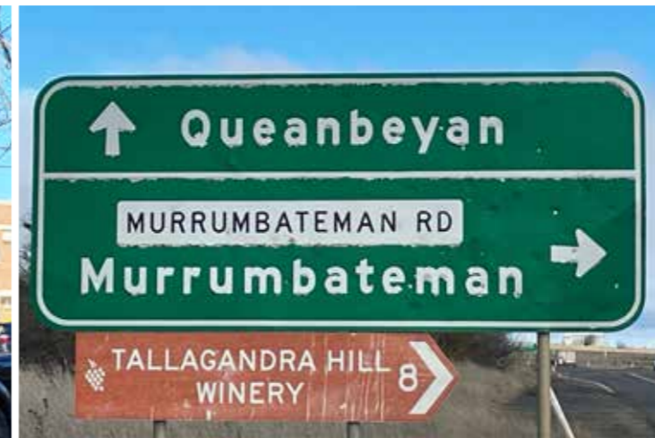
Sutton - The brown winery sign is an intersection sign, it should be an advance warning sign (see example page 14)
