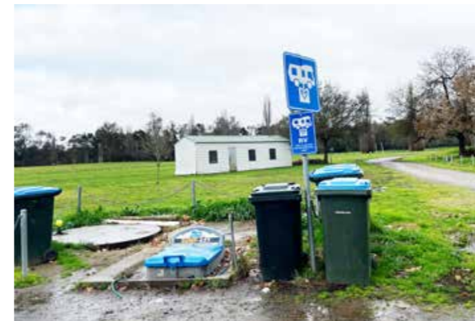
Jugiong RV dump point, no directional sign to this location from Riverside Dr. Dump point area needs to have a proper pad installed.
