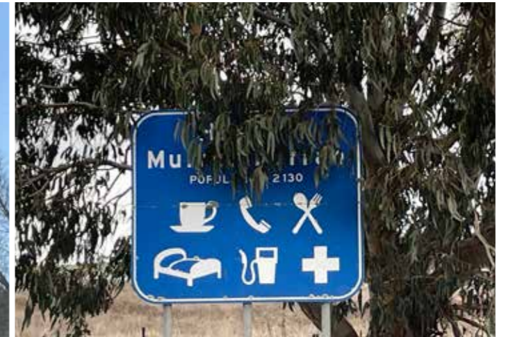
Harden - Advance warning signage overgrown
