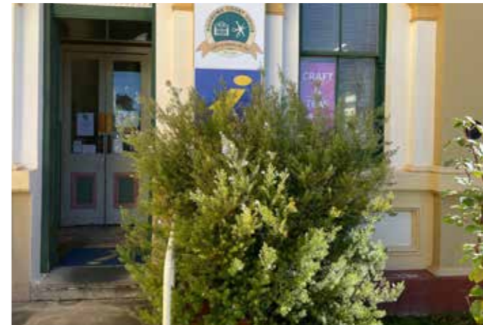
Boorowa Visitor Information Centre - Surely someone must have noticed that the main facility panel is becoming overgrown?
