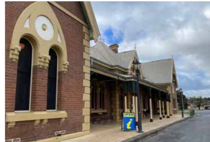
Young Visitor Information Centre - Due to the historical significance of the Young Train Station no substantial can be attached to the building
