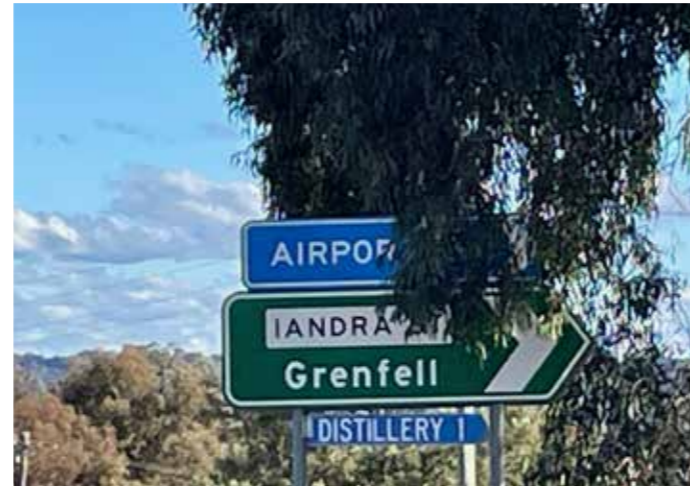
Young - Directional signage overgrown
