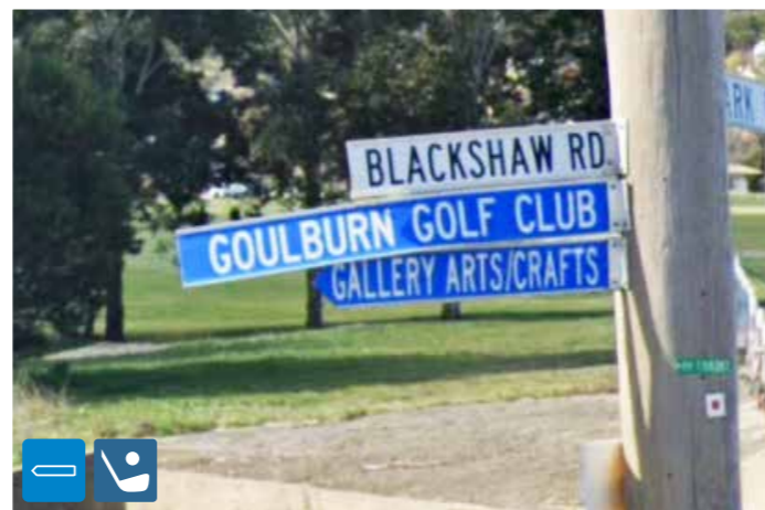
Goulburn - Damaged signage structure Blackshaw/Park Rd intersection.
