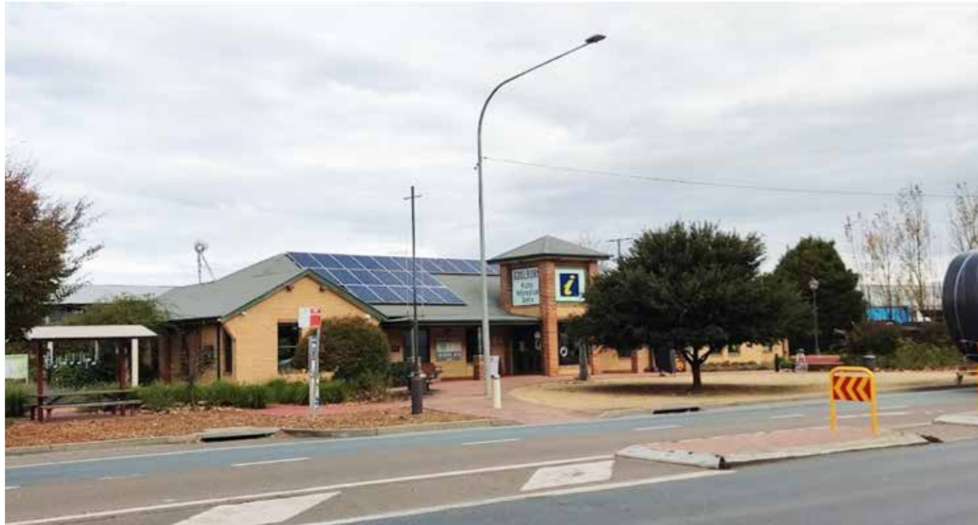
Goulburn Visitor Information Centre
